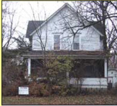
Before work began
