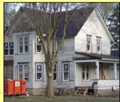
New windows are in
