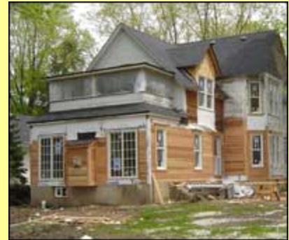
The rear of the house, with the sleeping porch above.
