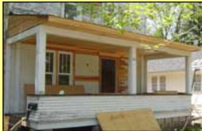
The front porch roof is rebuilt.
