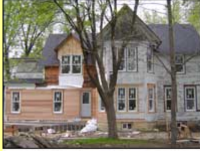
New siding on the south side of the house.
